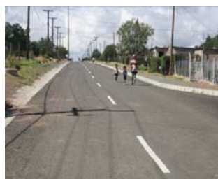
L Section: Bot Rd 551 – Project completed
