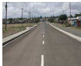
W Section: Project completed
